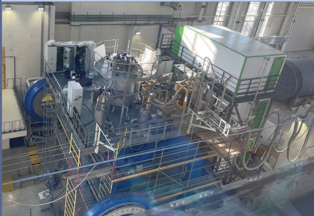
A general view of the technological platform of the MPD solenoid cryogenic cooling system with the equipment installed
